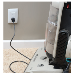
Wear and tear of appliance power cords can eventually lead to damaged conductors.
