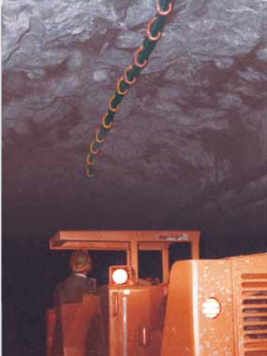
Bosserman Clips keep cables safely up and out of the way of moving equipment.
